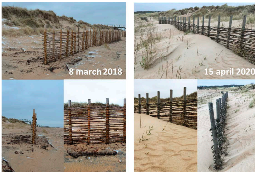
Comparison of sand accumulation and dune formation over the period 2018–2020 using sand fencing made of willow sticks at Vejbystrand in Ängelholm Municipality (pilot installation 25 metres long). Two years after implementation, significant amounts of sand had accumulated and vegetation was re-established. Photo and source: Anna Hamilton (2018) and Geraldine Thiere (2020). Illustration by GT.
