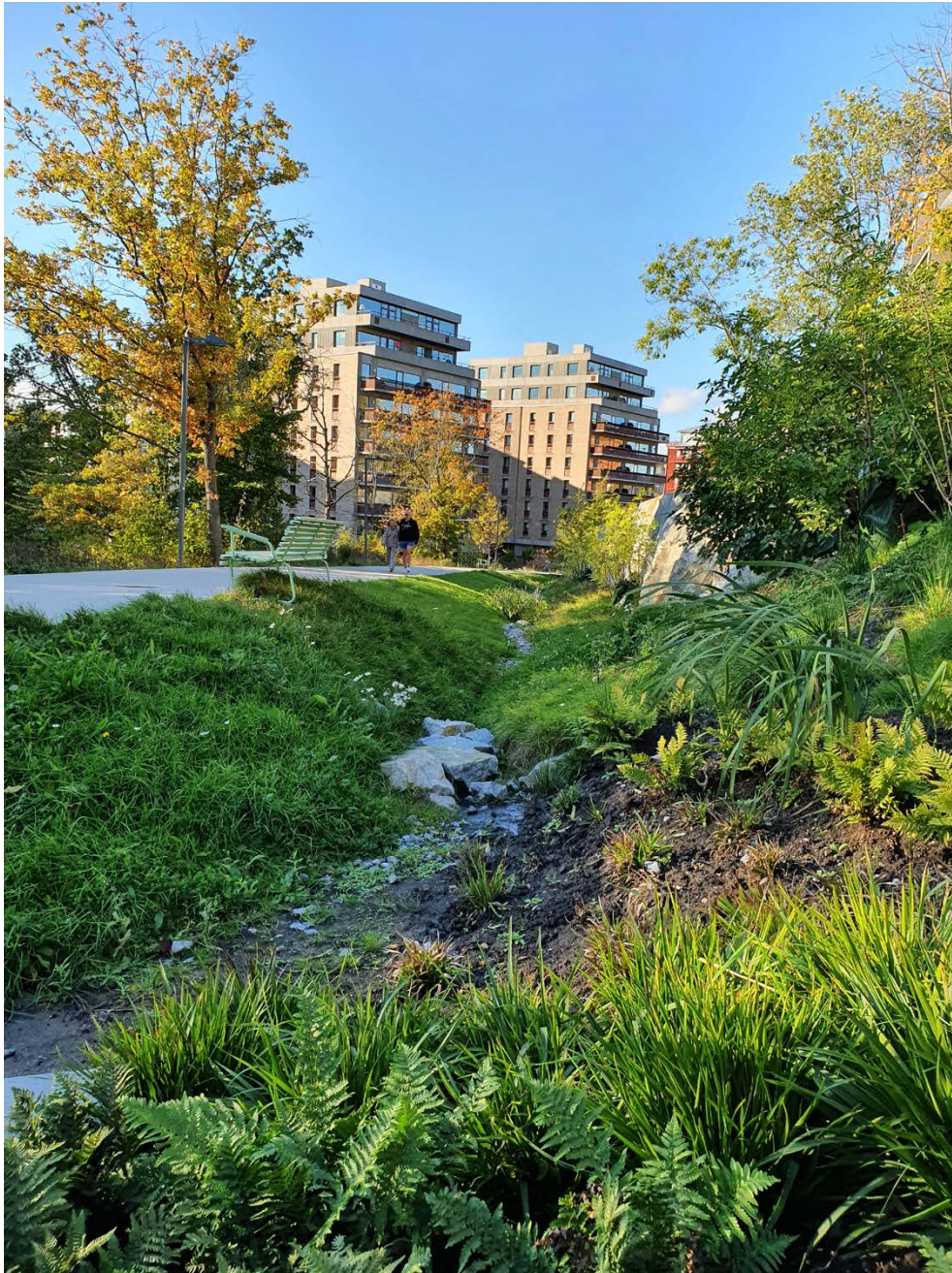
Swales and two-stage ditches are examples of open stormwater solutions that can be implemented to detain and divert stormwater during cloudbursts. At the same time, this type of nature-based solution can become a verdant recreational feature of the cityscape, as in this example from Norra Djurgårdsstaden in Stockholm. Photo: Timo Persson.
