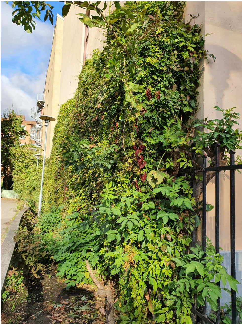
Green walls can become an attractive feature of the cityscape that promotes urban biodiversity, while helping to regulate temperature and manage stormwater. Photo: Timo Persson.
